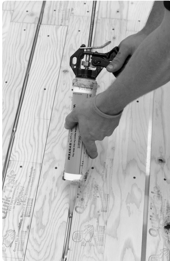
Figure 21: Insert a \frac{1}{8} " bead of sealant into the panel groove.
