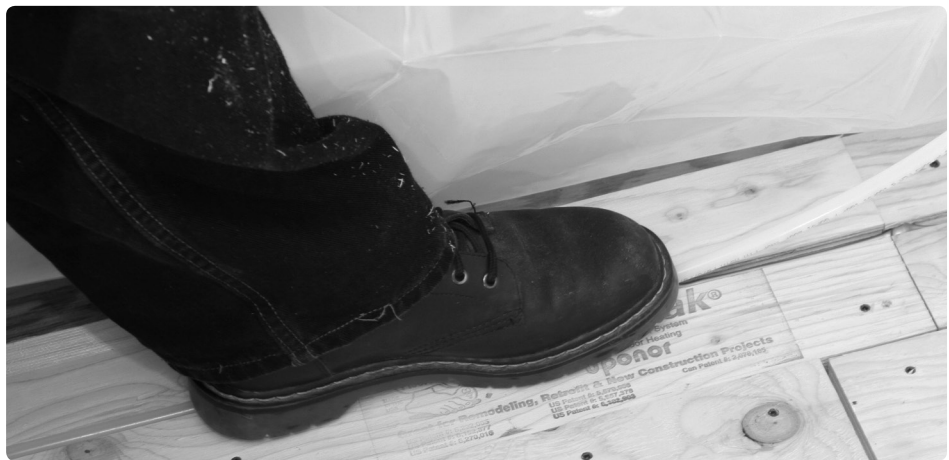
Figure 22: Use hard-soled boots or shoes to walk the tubing into the panel groove.
