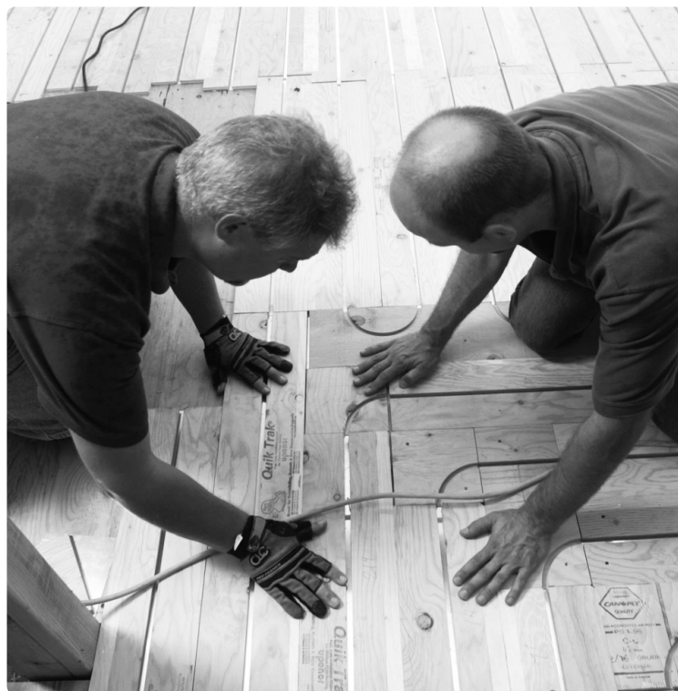
Figure 4: Installing Quik Trak Panels
