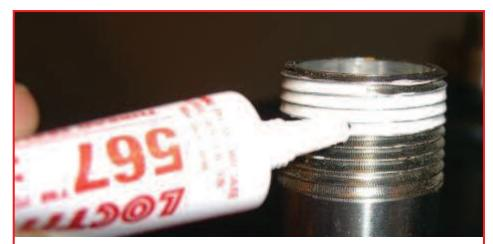
Only apply Loctite 567 in groove of male threads starting 1 thread from the end and continuing around the pipe 3 threads later on all appliance fittings/joints.
