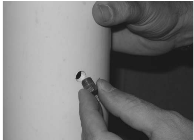
Figure 9.3: Insert Pipe Plug into Test Port
