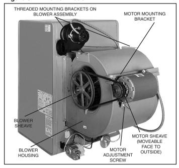
3. Adjust motor adjusting screw for a belt deflection of approximately 3/4" with five pounds of force applied midway between the sheaves (see Figure 9.3). Since the belt tension will decrease dramatically after an initial run-in period, it is necessary to periodically re-check the tension. Excessive tension will cause bearing wear and noise.
