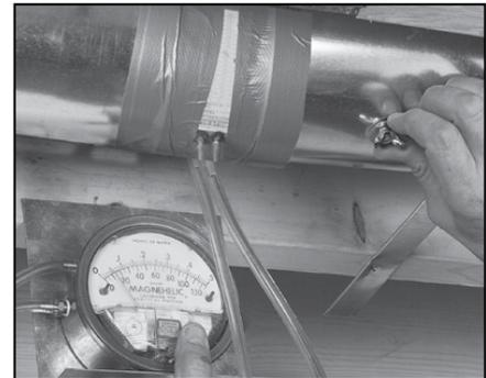
**3** Adjust the "Supply Air Out" damper until you reach the desired velocity. Follow the previous steps to adjust the "Exhaust Air Out" damper, if needed.
