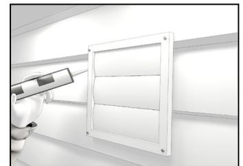
**4** Using a caulking gun, seal around both hoods to prevent any leaks.
