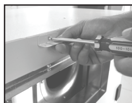
Figure 2 Support "A" installé
