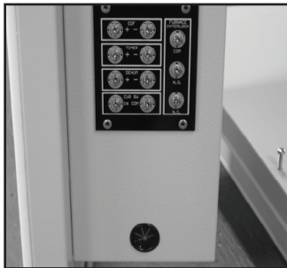
Figure 6 Insert damper motor wires through bushing
