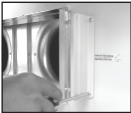
Figure 1 Bracket "B" Installed
