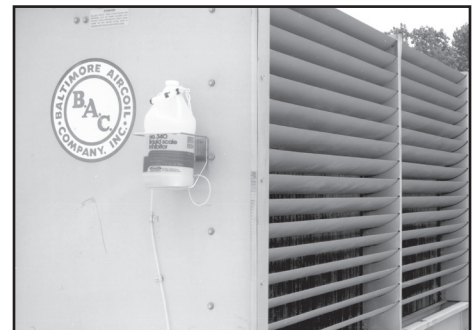
Arrange Drip Feeder so that weighted end is proper distance above or below surface of sump water.
