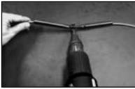
**Step 2.18.** Slide the outer shrink tube over the entire connection, centering it. Use a heat gun to shrink the tube, beginning near the middle, moving back and forth until it is fully shrunk down. Do not over heat the tube or the heating cable jacket, causing damage. Allow to cool.
