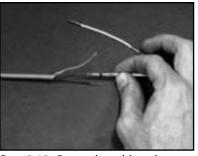
**Step 2.12.** Center the solder tube over the twisted connection. Make sure the stripped wires are fully between the **gray** adhesive bands at the ends of the solder tube. If this is not done, the wires may pull out or water may enter this connection causing failure.
