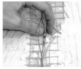
**Step 3.13.** Pull the heating wires together to overlap the heating elements of both leads. Lightly twist the elements together to better join them. Slide the solder tube over the twisted elements, centering the elements between the gray adhesive bands. If this is not done correctly, the elements may pull out and cause the splice to fail.
