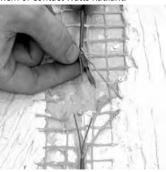
**Step 3.12.** Slide the solder tube over one of the heating wires.
