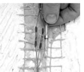
**Step 3.16.** Slide a ground solder tube over a ground braid lead. Overlap the braid ends and twist them to help hold them together. Slide the ground solder tube over the twisted braid ends, centering them under the ring of solder.
