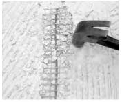
Step 2.2. Remove enough mortar and tile to expose about 4" to 5" of free wire on both sides of the damaged portion. Part of the wire may be visible so that the mortar can be removed carefully around the damaged wire using the hammer and/or chisel. Mesh can be cut with scissors in order to free the wire.
