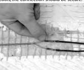
**Step 4.21.** At the other end of the ground jumper wire, slide a ground solder tube over the wire. REPEAT Step 4.20 to complete this connection. Be sure to avoid reheating or scorching the heating wires or splices, using a heat shield again if needed.
