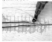
**Step 4.20.** Overlap the ends of a ground braid lead and the ground jumper wire by about 1/2" and twist them together. Slide a ground solder tube over the twisted ends, centering the ends under the solder ring. Heat the tube to shrink it completely and cause the solder to flow into the wires completely. Be sure to avoid reheating or scorching the heating wires or splices, using a heat shield like a wet cotton rag or a piece of tin if needed. When it cools, the connection should be secure.
