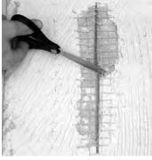
Step 3.1. Cut out the damaged wire location, creating two ends or leads. If the cable being repaired is not the jacketed heating cable, skip to Step 3.6.
