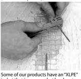
some or our products have an "XLPE" jacket that is a somewhat hard material that can be lightly "scored" with a scoring tool or sharp blade. Use the scoring tool to carefully score the jacket about 2.5" from the end of each lead. Do this by placing the cable lead into the V-notch of the tool and rotating the tool only one or two revolutions around the cable. Do not place any additional pressure on the tool head to cut deeper. Let the tool apply its own spring-loaded pressure.
