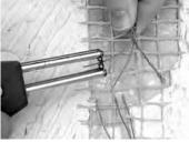
**Step 3.10.** Use the thermal wire strippers to carefully strip off exactly 1/2" of the insulation from the heating wires. Count the little heating elements to make sure none were cut off and thereby cause a hot spot or possible failure. A fiber strand may also be found among the heating elements. There is no need to separate or remove this fiber strand.
