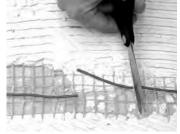
**Step 4.1.** Cut out a 2"- to 3"-long section of the heating cable around the damaged area, creating two ends or leads.
