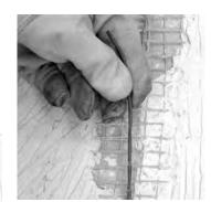
**Step 3.5.** Use a glove or other protective cloth to pull off the loosened jacket slug. **Do not touch** the hot jacket slug with bare fingers. The slug will be very hot and will burn!
