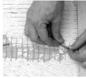
**Step 4.3.** Gently bend the cable at the score to break through the jacket all the way around the cable, then pull off the slug.
