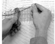
Some of our products have an "XLPE" jacket that is a somewhat hard material that can be lightly "scored" with a scoring tool or sharp blade. Use the scoring tool to carefully score the jacket about 2.5" from the end of each lead. Do this by placing the cable lead into the V-notch of the tool and rotating the tool only one or two revolutions around the cable. Do not place any additional pressure on the tool head to cut deeper. Let the tool apply its own spring-loaded pressure.
