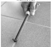
**Step 2.1.** If not done so already, carefully remove the tile/stone/marble floor covering over the damaged cable area. Removal of the grout around the affected tile(s) must be done with a blunt instrument such as a hand-held grout-removal tool. **DO NOT USE A KNIFE!** Gently break out the tile with a small hammer, removing the fragments as the tile is broken up. See wattsradiant.com for additional instructions and tips regarding tile removal.
