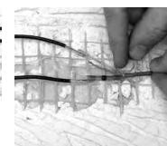
**Step 4.18.** At the other end of the jumper wires, slide a heating element solder tube over a heating wire or its jumper wire, which ever is easier for you to position the tube out of the way and allow for easy access to the ends of the wires. REPEAT Steps 4.14 through 4.17 to complete the heating element jumper wire connections.
