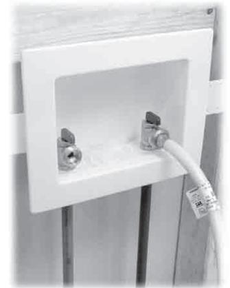
Dual-valve washing machine enclosure with 1/2" (15mm) CrimpRing™ fittings and flexible PVC supply lines.
