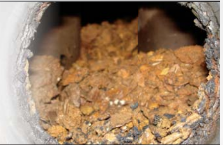
“In-tank” flue tubes and heat exchangers suffer from lime scale buildup beginning from the first hours of operation.
