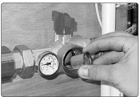
**Step 5**Remove any dirt and debris from the filter.
