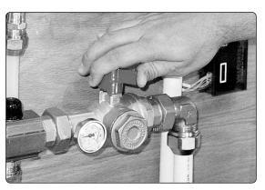
**Step 3**Remove the circlip which retains the filter.
