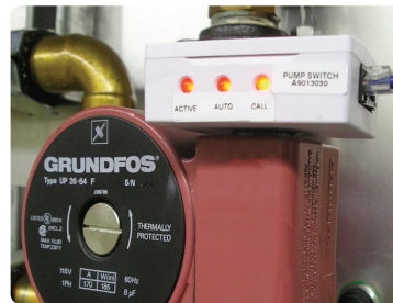
Figure 1: Pump Mounting
