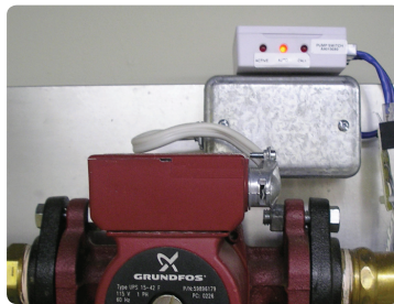
Figure 2: Electrical Box Mounting
