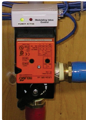
Figure 1: Belimo Valve Mounting
