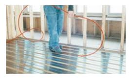
RAUPANEL is a great option for retrofit and new construction applications because it is installed without the concrete overpour. RAUPANEL can work with all types of flooring.
