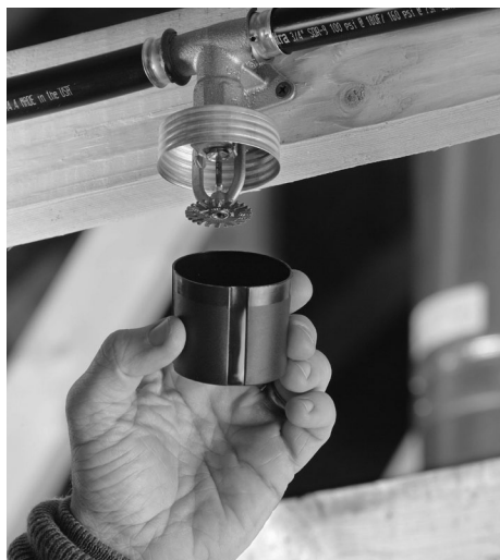
Keep heads within protective shell during installation
