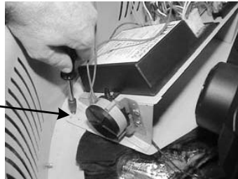
Control Panel Mounting Screw
