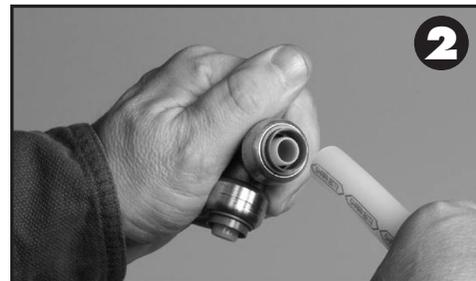
**Step 3.** Insert the tube into the fitting until the tube reaches the tube stop. Make sure the pointed end of the SharkBite pattern is even with the end of the release collar. Only when the tube reaches the tube stop has a secure joint been created.
