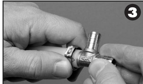
**Step 4.** Position the open jaws of the clamp tool over the raised tabs of the clamp ring and squeeze.
