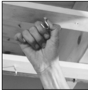
1 Place Fastening hooks on the strapping board or the floor joists.
