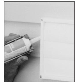
**4** Using a caulking gun, seal around both hoods to prevent any leaks.
