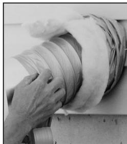
**2** Pull the insulated flexible duct through the opening until it is well extended and straight. Slide the duct's inner vinyl sleeve over the hood collar and secure. Pull the insulation over the sleeve. Secure with duct tape.
