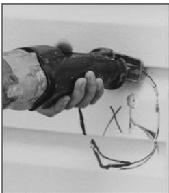
**1** Using the collar of the outside hood, outline the intake & exhaust hole to be cut. The holes should be slightly larger than the collar to allow for the thickness of the insulated flexible duct. Cut a hole for both the intake and exhaust hoods.
