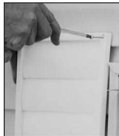
**3** Push the hood into the opening, then attach the hood to the outside wall with mounting screws. Repeat the installation procedure for both the Supply and Exhaust hoods.
