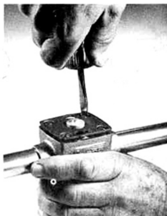
2—Remove the 4 Screws from hold down plate
