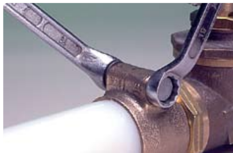
8. Tighten the Fitting
